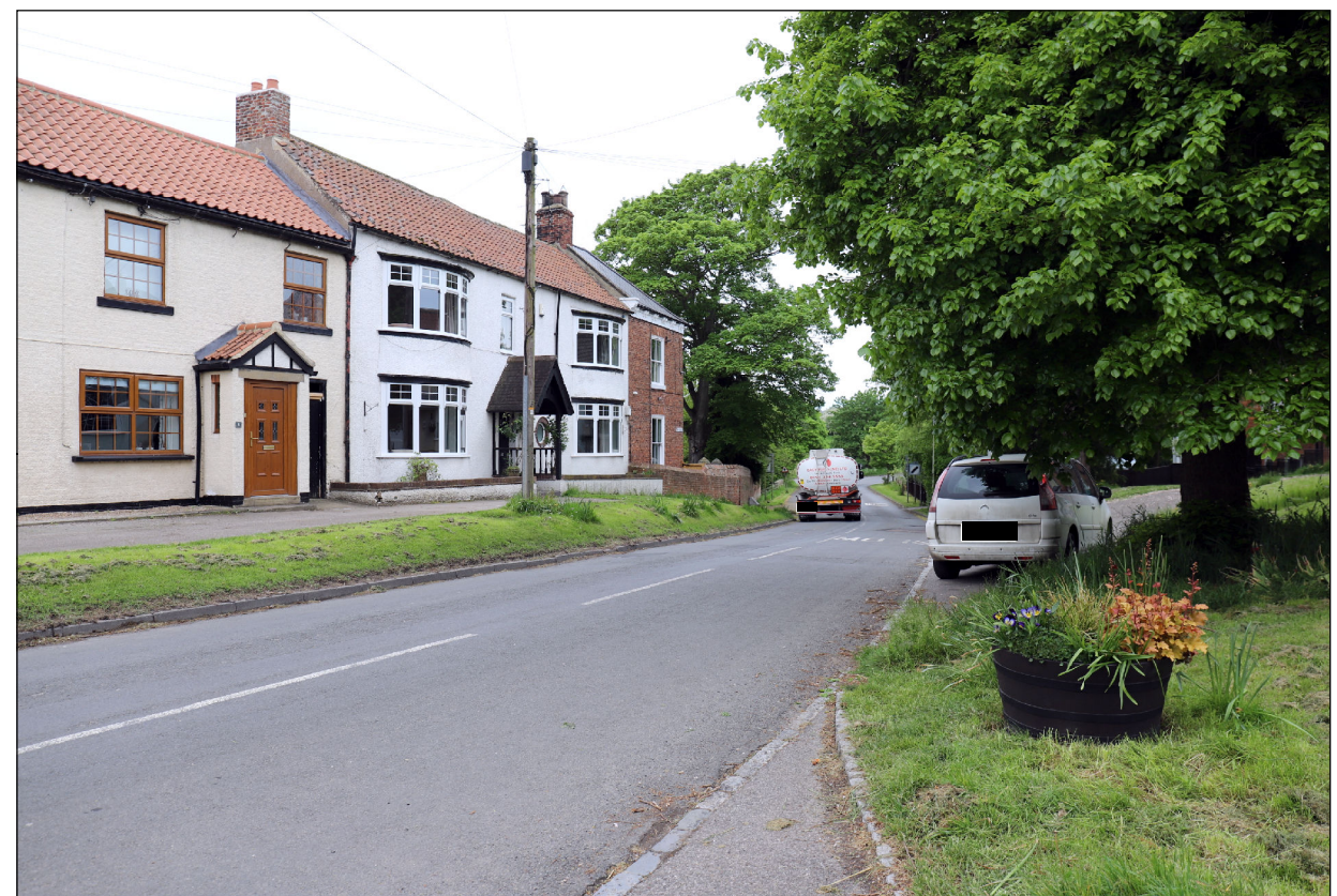
Plate 50) View along Bishopton High Street looking northwest
