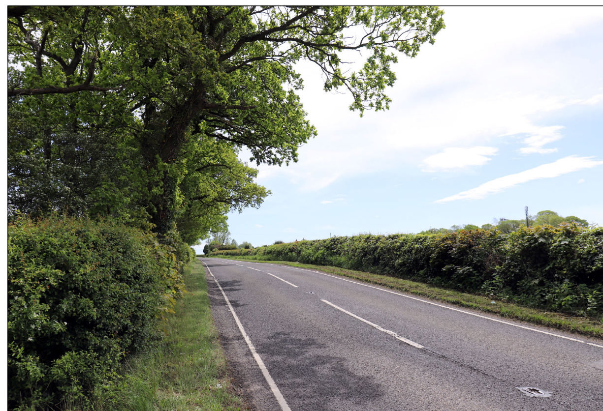
Plate 54) View of earthworks from Whitton Road, looking east
